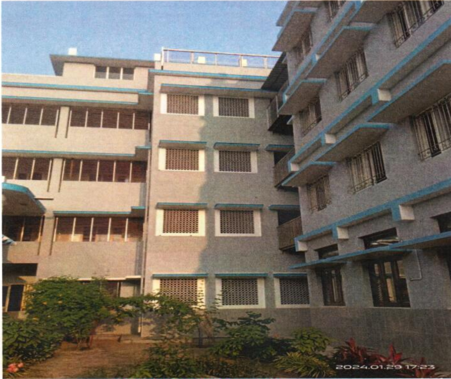
TOILET BLOCK IN KG BUILDING
