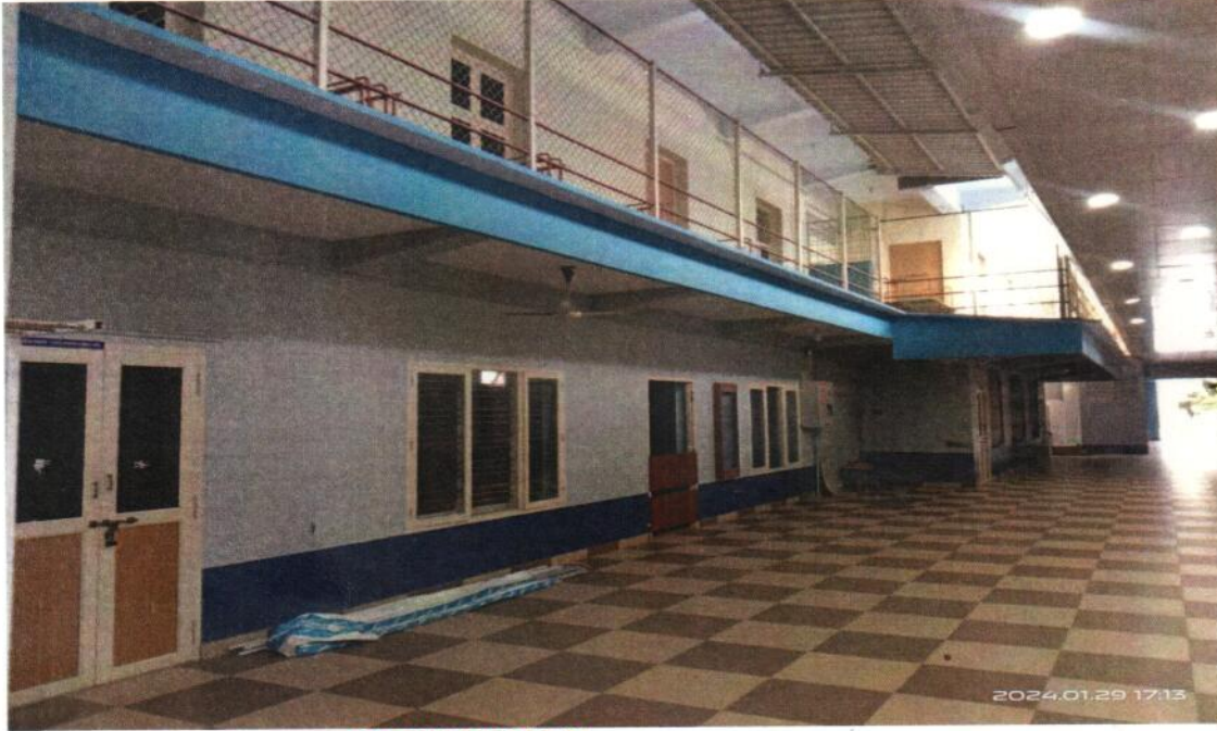
OLD BUILDING [G+2]
